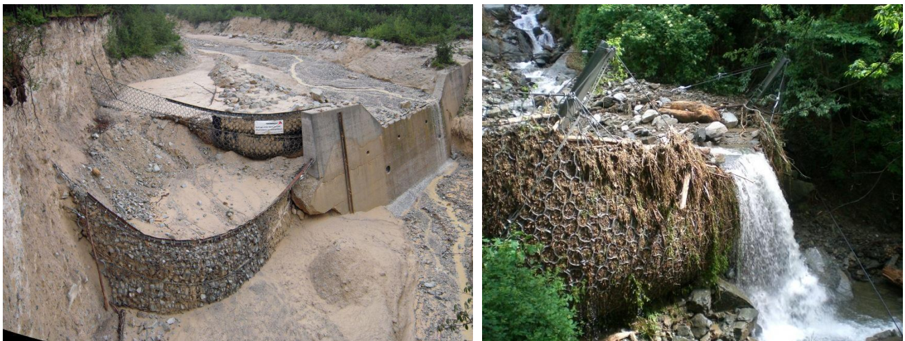
Figure 1: Application of ring net barriers as an additional building to a concrete check dam in the Illgraben in Canton Valais in Switzerland (left) and a successfully filled ring net barrier in Italy (right).
