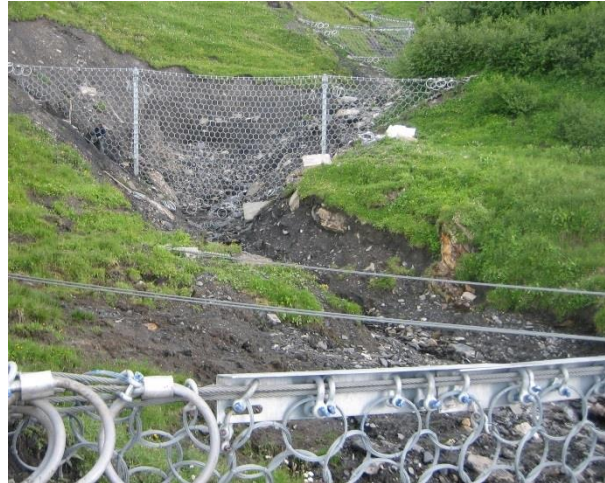
Figure 3: Multilevel barriers in the Hasliberg region in the Bernese Alps.
